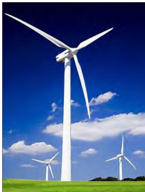
A wind turbine may contain 335 tons of steel, 4.7 tons of copper, 13 tons of fiberglass, 3 tons of aluminum and 1,200 tons of reinforced concrete.
