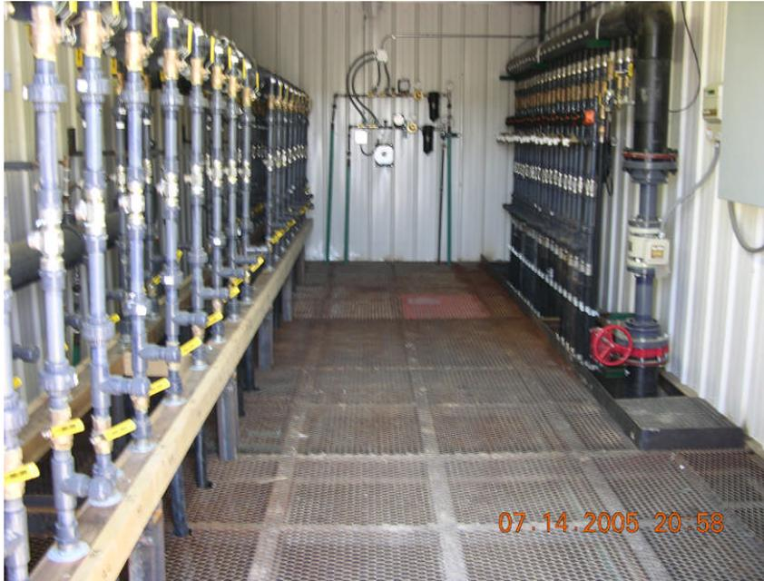
Header House, controlling both injection as well as production from many wells in wellfield
