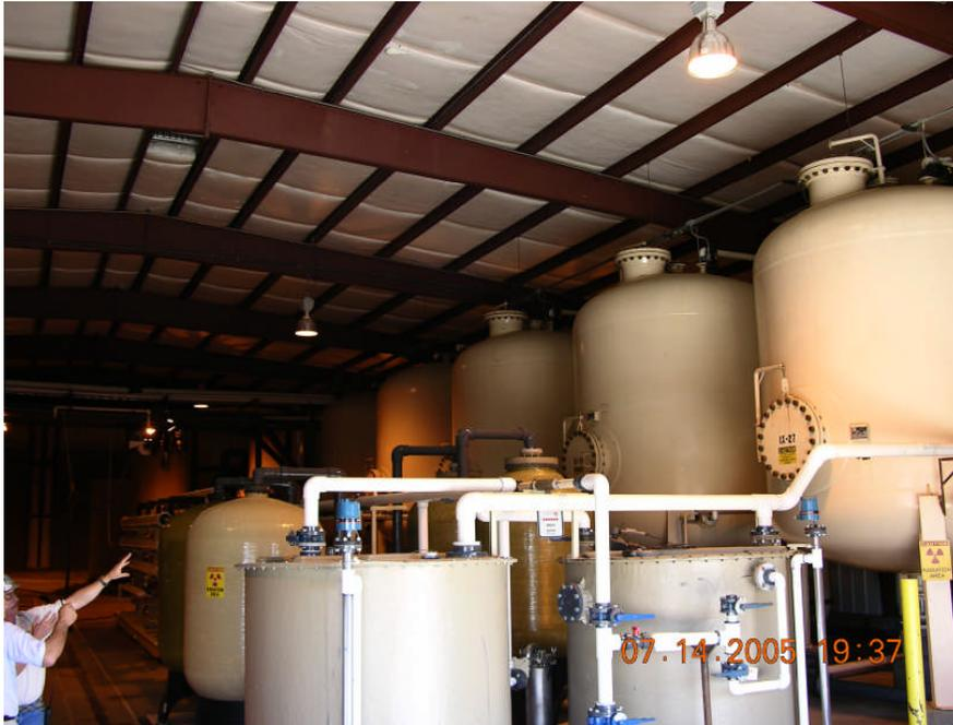
From the production well the produced fluid goes through resin tanks where the uranium is stripped from the fluid and is then returned to the wellfield
